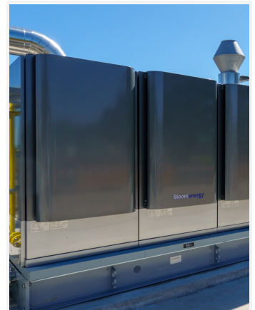
© EnBW Energie Baden-Württemberg AG.
