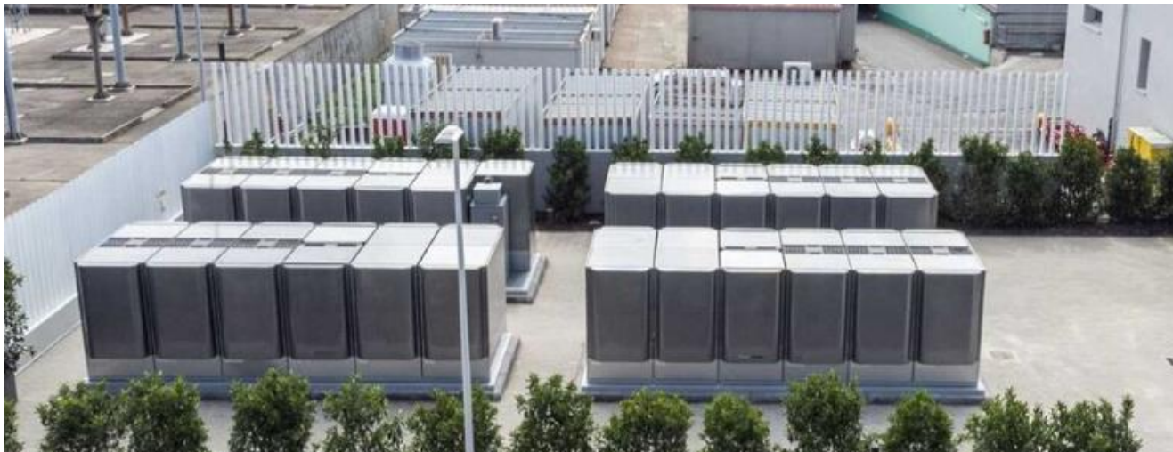
1 MW Energy Server installation at the Ferrari HQ in Maranello (front view)
